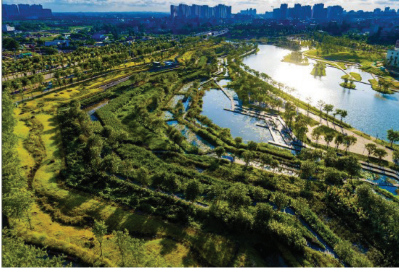
FIGURE 4-2 Constructed wetlands to cleanse contaminated water, Haikou Meishe River, Hainan, China.
