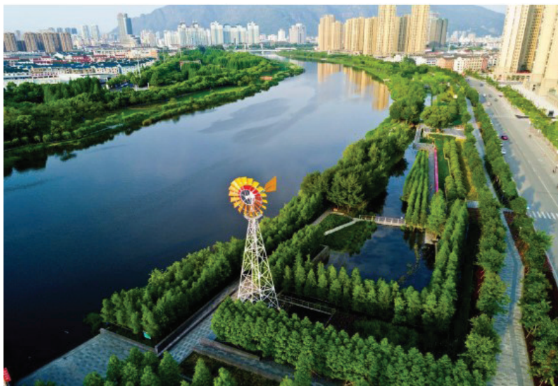
FIGURE 4-1 Use of a resilient ecological embankment to replace the former concrete flood control infrastructure, Yongning River, Taizhou, Zhejiang.
